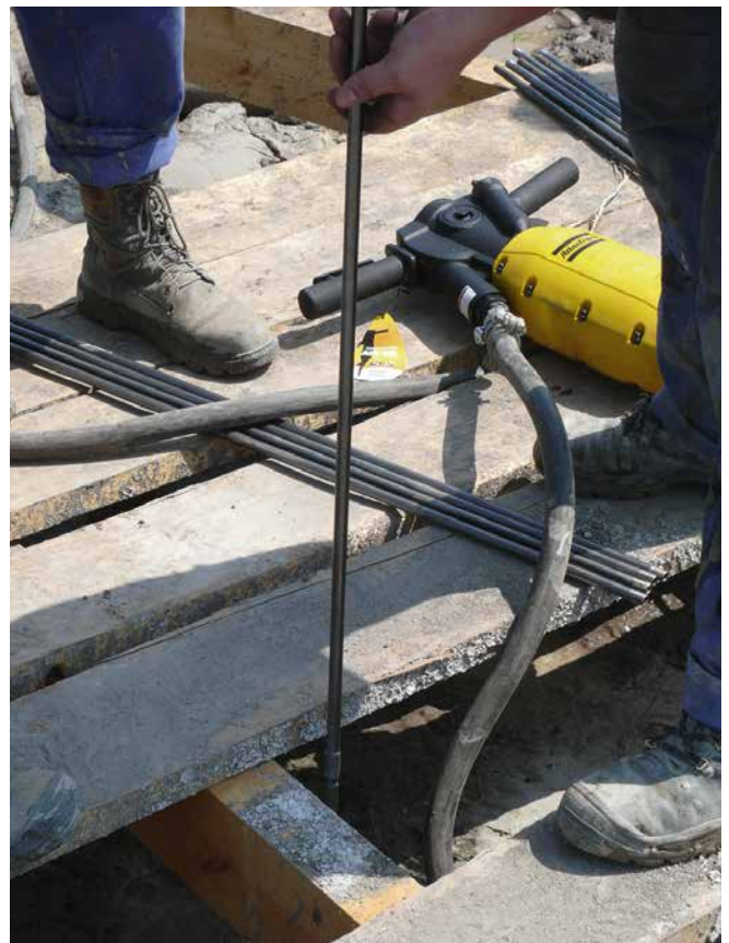
Introduction of the ram injection lances (photos: Desoi)
