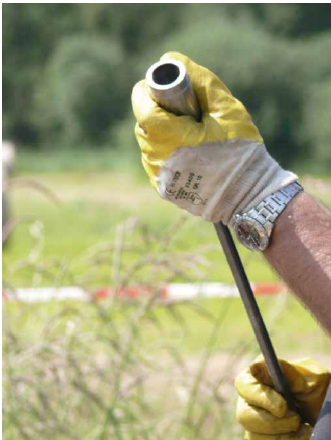
Installation of ram injection lances
